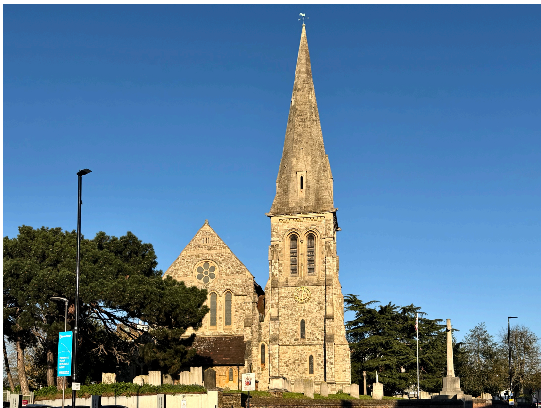
The Church Built on a Hill
